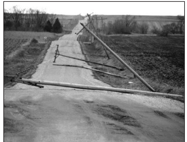
Several poles down from tornadoes.
