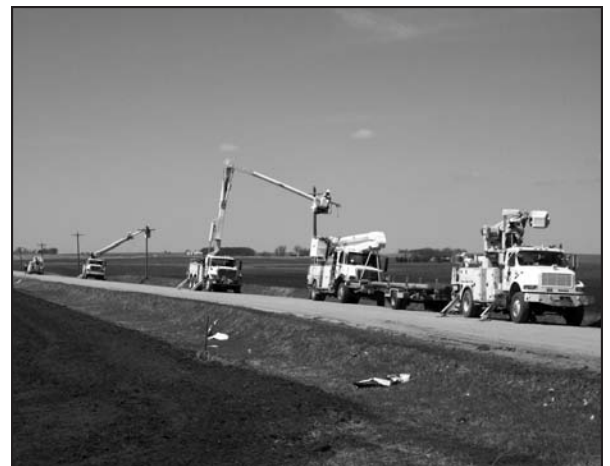
Line crews making repairs.
