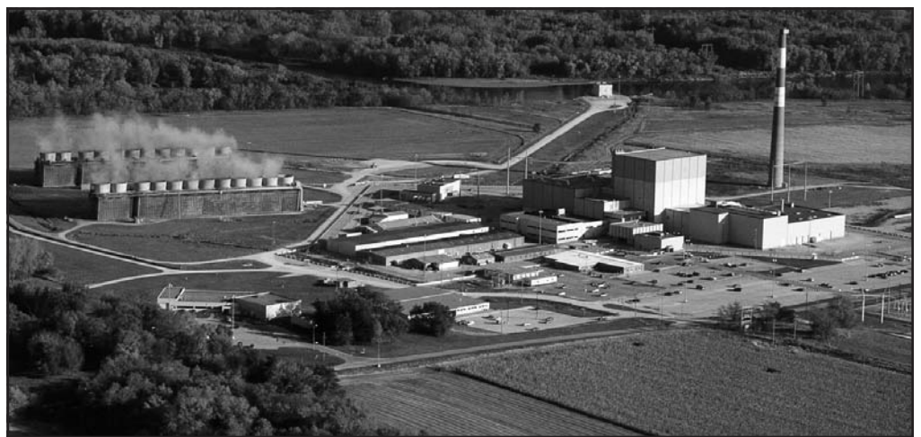
Duane Arnold Energy Center – Iowa's only nuclear power plant – received a 20-year license extension from the Nuclear Regulatory Commission Dec. 16. Corn Belt Power Cooperative, wholesale power supplier to Raccoon Valley Electric Cooperative, owns a 10 percent share of the plant, located near Palo, Iowa.
