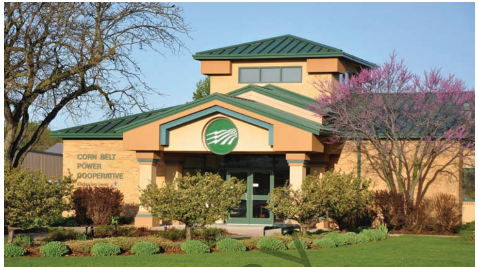
Corn Belt Power Cooperative located in Humboldt, Iowa.
