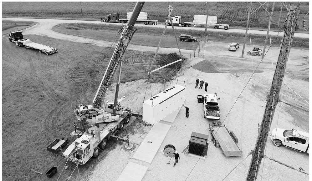
Corn Belt Power’s utility scale battery storage installation at the Hampton Substation.
